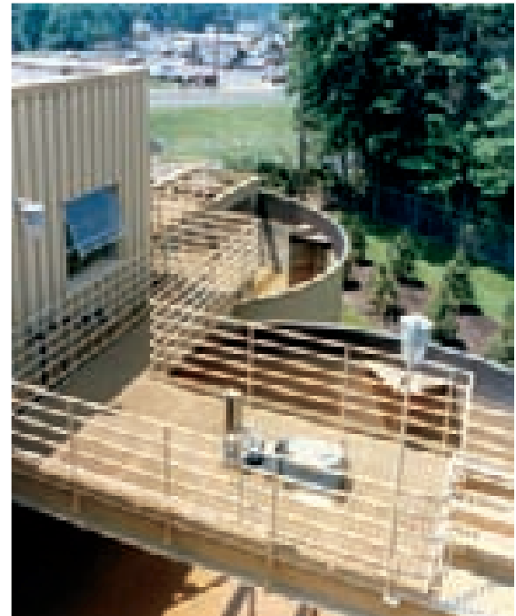
1984 WASTEWATER TREATMENT FACILITY, FORD MOTOR COMPANY Edison, New Jersey Architect: Samborn, Steketee, Otis & Evans, Inc.
