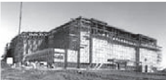
The Macy's featured to the right under construction
