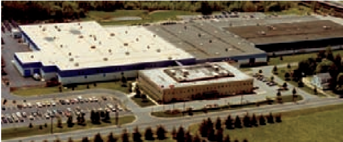
1983 MANUFACTURING ADDITION, LANGSTON, A DIVISION OF MOLINS MACHINE COMPANY Cherry Hill, New Jersey • Architect: Hill Associates
