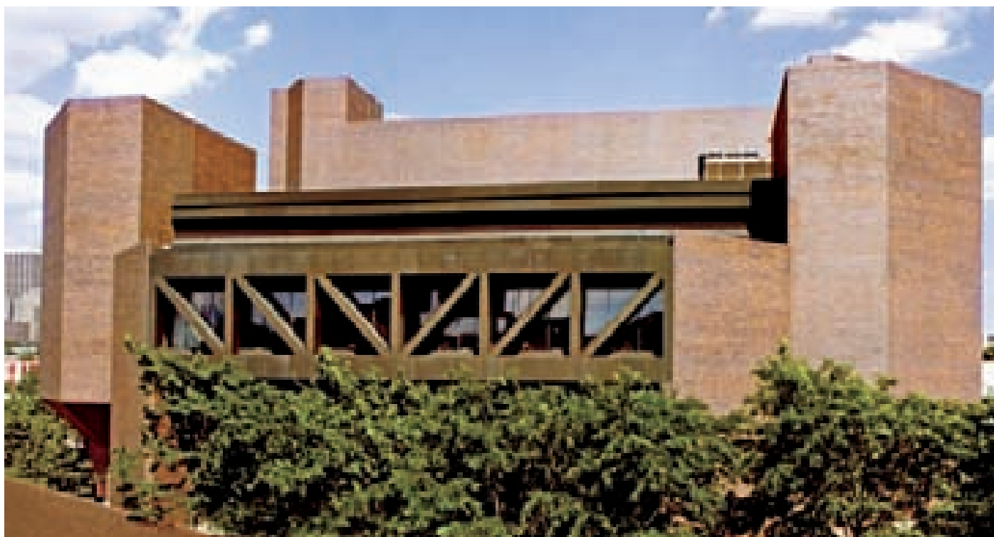
1971 ▼ TELEPHONE EXCHANGE BUILDING, BELL TELEPHONE COMPANY OF PENNSYLVANIA
