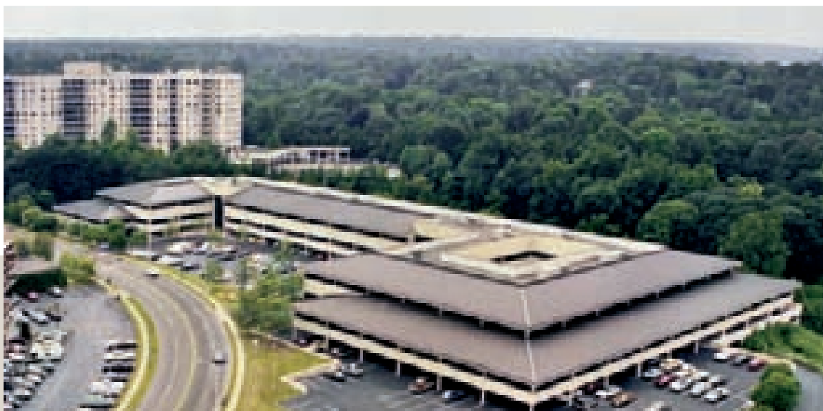
1973 CORPORATE OFFICE BUILDING, HONEYWELL, INC.
