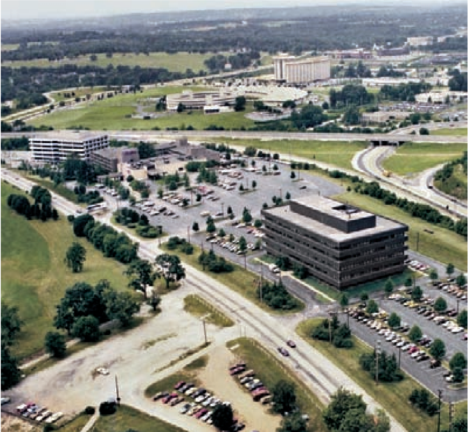
1979 ▼ THE LEIGHTON BUILDING, STOFFER'S HOTEL AND THE IRWIN BUILDING King of Prussia, Pennsylvania
