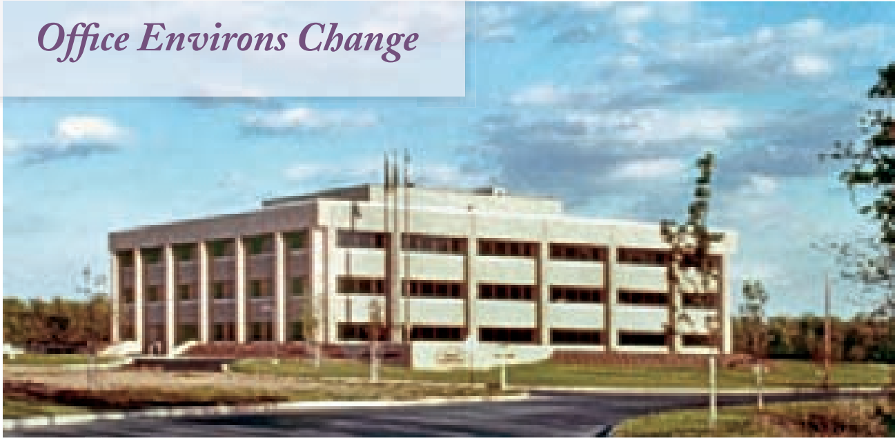
1976 REGIONAL HEADQUARTERS OFFICE BUILDING, UNION CARBIDE CORPORATION
