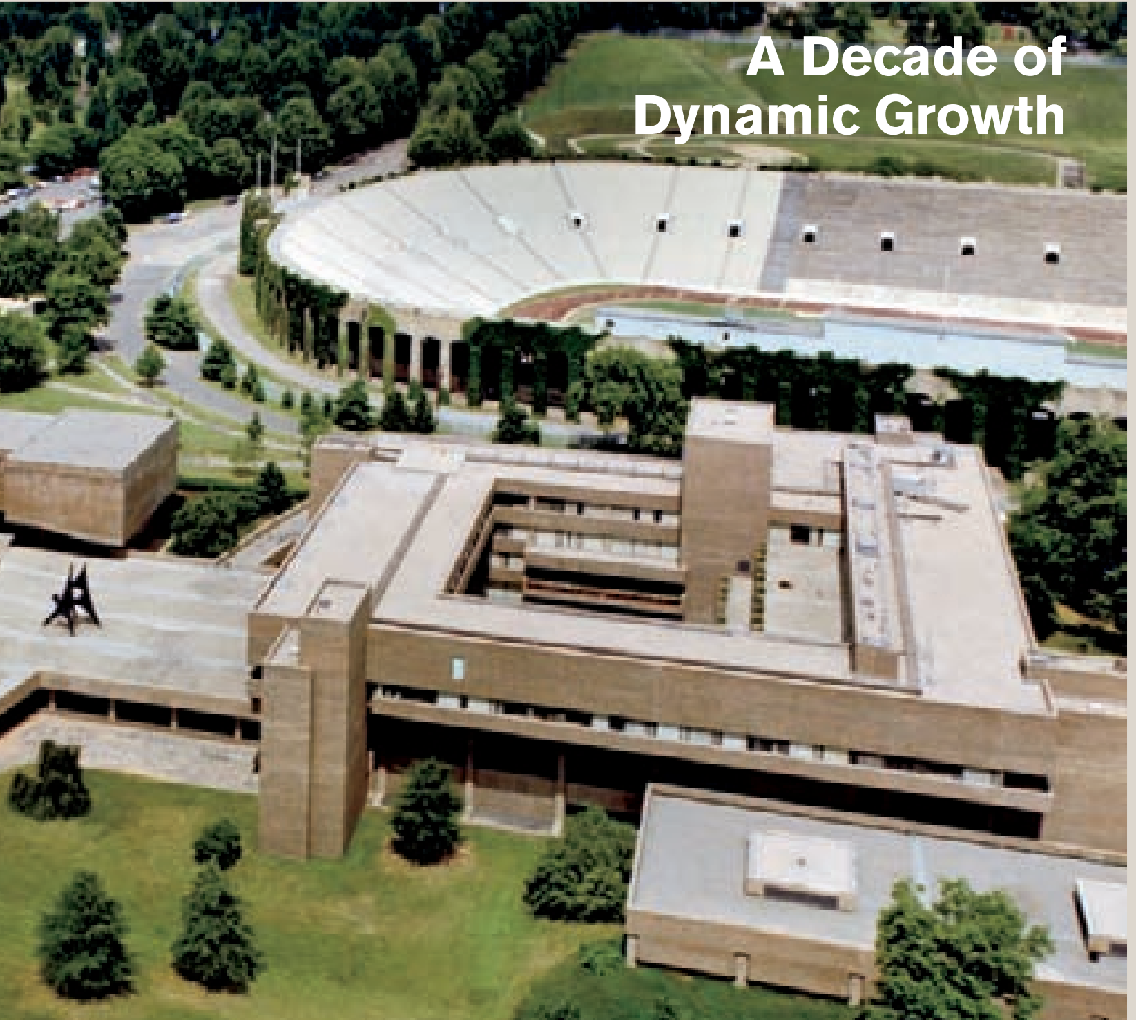
1970 MATHEMATICS-PHYSICS COMPLEX, PRINCETON UNIVERSITY Princeton, New Jersey • Architect for Fine Hall: Hugh Stubbins and Associates Architect for Jadwin Hall: Warner Burns Toan & Lunde
